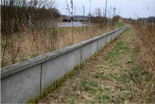
Synthetic amphibian fences tend to show failures a few years after installation (top). Concrete barriers are a sustainable alternative (bottom).
